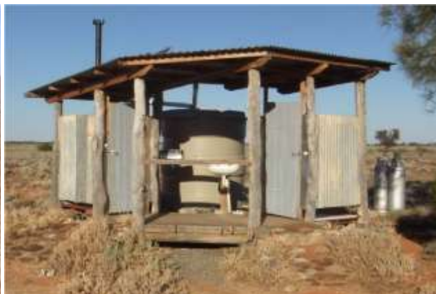
Boolcoomatta bush campground with hot and cold showers using roof runoff and groundwater Date 20170414 N° 8038 Photo DM Trebilcock
