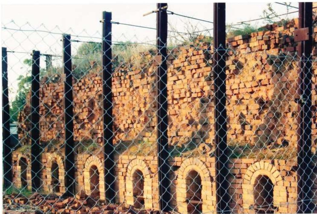
Crumbling brickwork of kiln with fallen bricks scattered at base.
