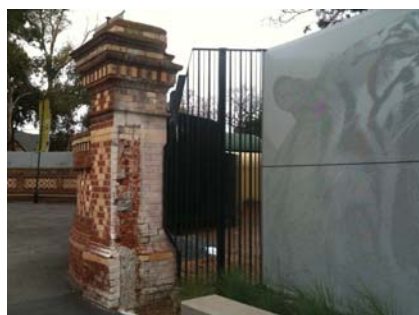
Condition of heritage column
