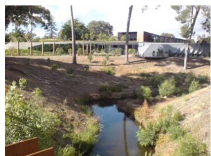
New entrance from Frome Road at bridge
